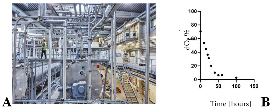
Figure 1: Photo from the saccharification section at Meliora Bio and graph showing abiotic oxygen consumption at 50°C in a sample of the liquified wheat straw slurry taken during production.
